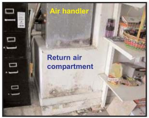
This photo shows a problem air-handler in a garage. A cabinet up against the AC unit base (return air plenum) hid the mold and water stains from sight. Everyone in the house was sick. The inside of the AC return air compartment was black with toxic mold. This was easily replaced with new by the AC service. Within weeks, everyone returned to health without the need for toxinbinding therapy.
