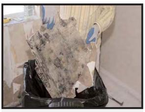
Hidden mold may be extensive even though only a slight glimpse is indicated on the outer wall. This was caused by a leaking sink. Indoor levels of toxic mold were **100,000** times higher than the outdoor levels.
