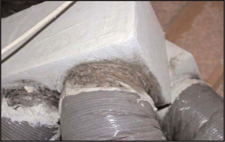
A duct leak in the attic caused this mold growth. The residents inside were getting sick because the hatch to the attic did not close well. If the house is properly sealed from the attic, moderate mold growth in the attic usually will not make people inside the home sick.
