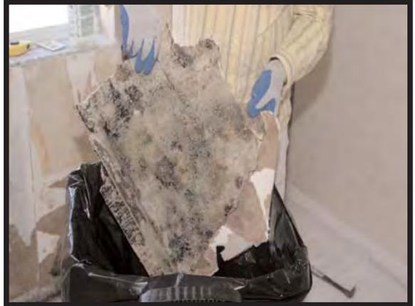
Hidden mold may be extensive even though only a slight glimpse is indicated on the outer wall. This was caused by a leaking sink. Indoor levels of toxic mold were **100,000** times higher than the outdoor levels.
