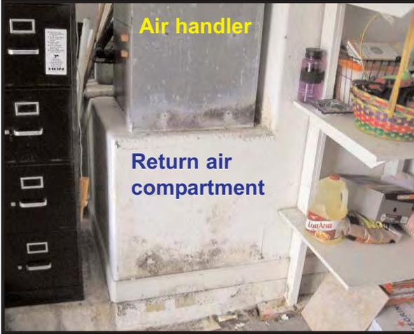
This photo shows a problem air-handler in a garage. A cabinet up against the AC unit base (return air plenum) hid the mold and water stains from sight. Everyone in the house was sick. The inside of the AC return air compartment was black with toxic mold. This was easily replaced with new by the AC service. Within weeks, everyone returned to health without the need for toxin-binding therapy.
